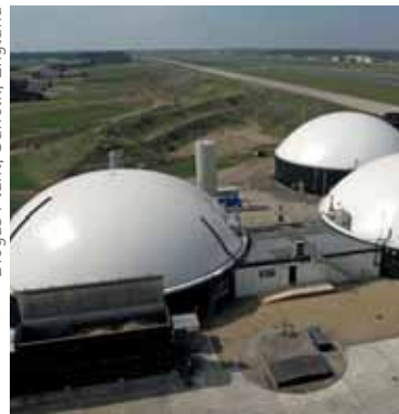
Biogas Plant, Suffolk, England
